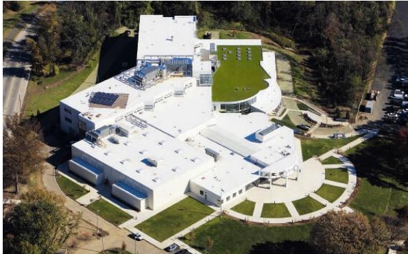
Fig.3: White colored Cool Roof in USA [5]
