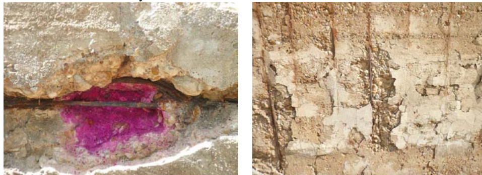
Figure 2: Deterioration of concretes in sewage treatment plant [16]
